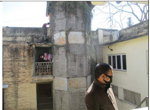
Vulnerable building attached to the lab building
