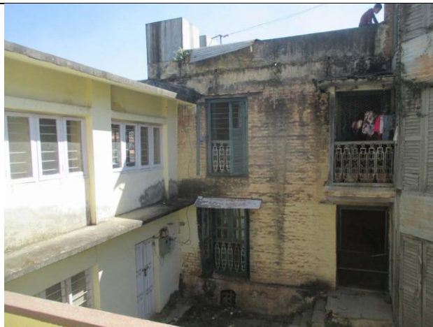
Vulnerable building attached to the lab building
