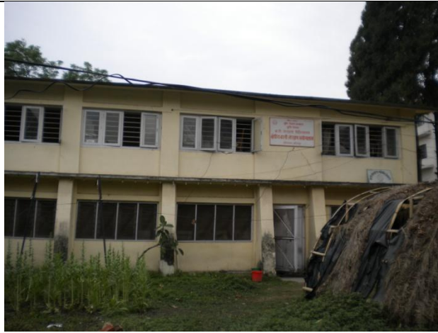
existing open space and front view of the building
